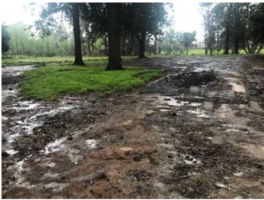
Photograph 3. Internal road north, looking east.
