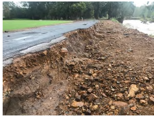
Photograph 4. Internal road and previous location of pathway, which was located at the same grade of the road.
